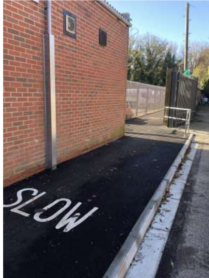
Widened link to NCN23 for cycles
