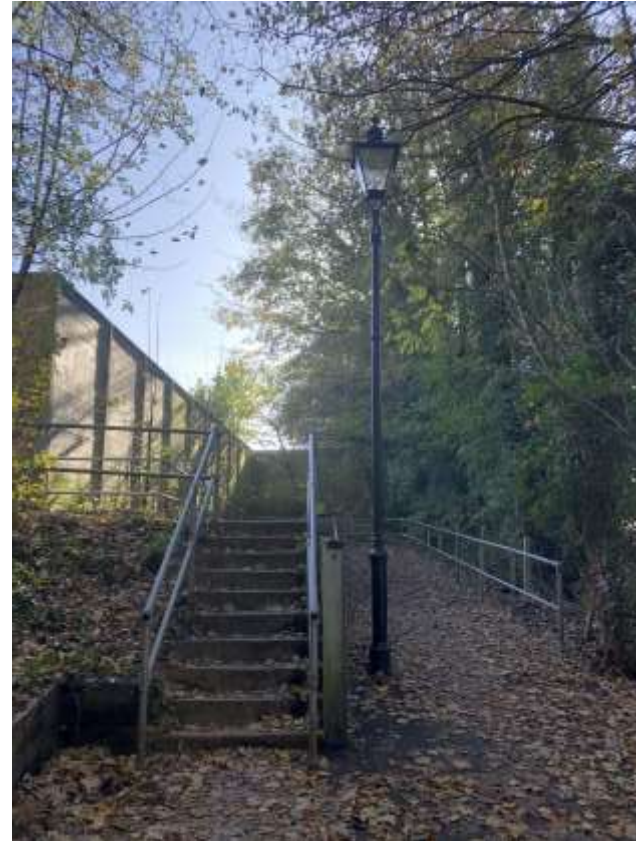
New street lighting along Domum Road
